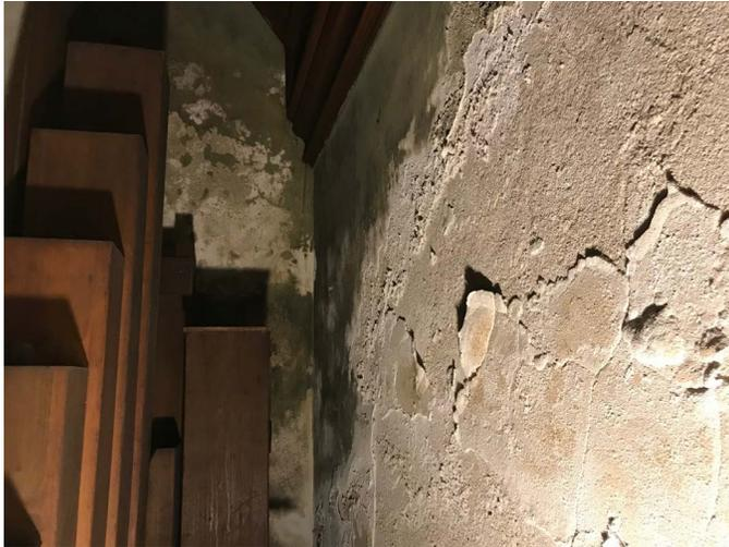
*Wooden bass pipes; scaling, water-damaged chamber walls*
